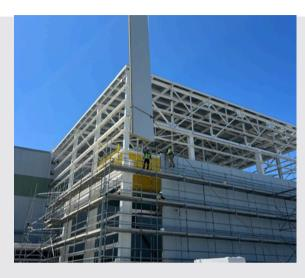
Paper Mill - Skowhegan, Maine Scaffolding erection and metal siding installation for a paper machine
