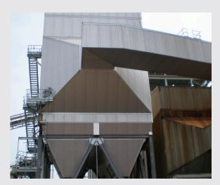
Paper Mill - Pine Hill, Alabama Completed industrial metal siding around precipitator with scaffold erection and dismantle
