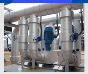
**Power Plant - Bridgeport, TX**Insulated metal pipe lagging for power plant industrial piping
