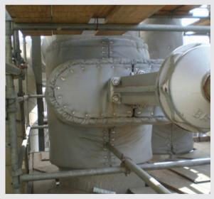
**Power Plant - Bridgeport, TX**Insulation blankets made and installed around industrial pipe
