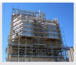
**Paper Mill - Valdosta, Georgia**Industrial scaffold erected to provide insulation and lagging for precipitator
